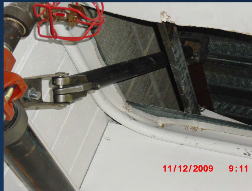
Ben Boeke Ice Arena Anchorage Wall/Roof Seismic Reinforcements 2009
