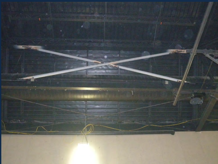
Kodiak Island Borough School District Seismic Roof Bracing Improvements 2011
