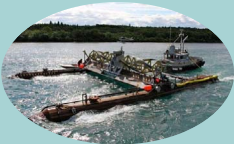
Igiguig hydrokinetic power (Ocean Renewable Power Co.) 1
