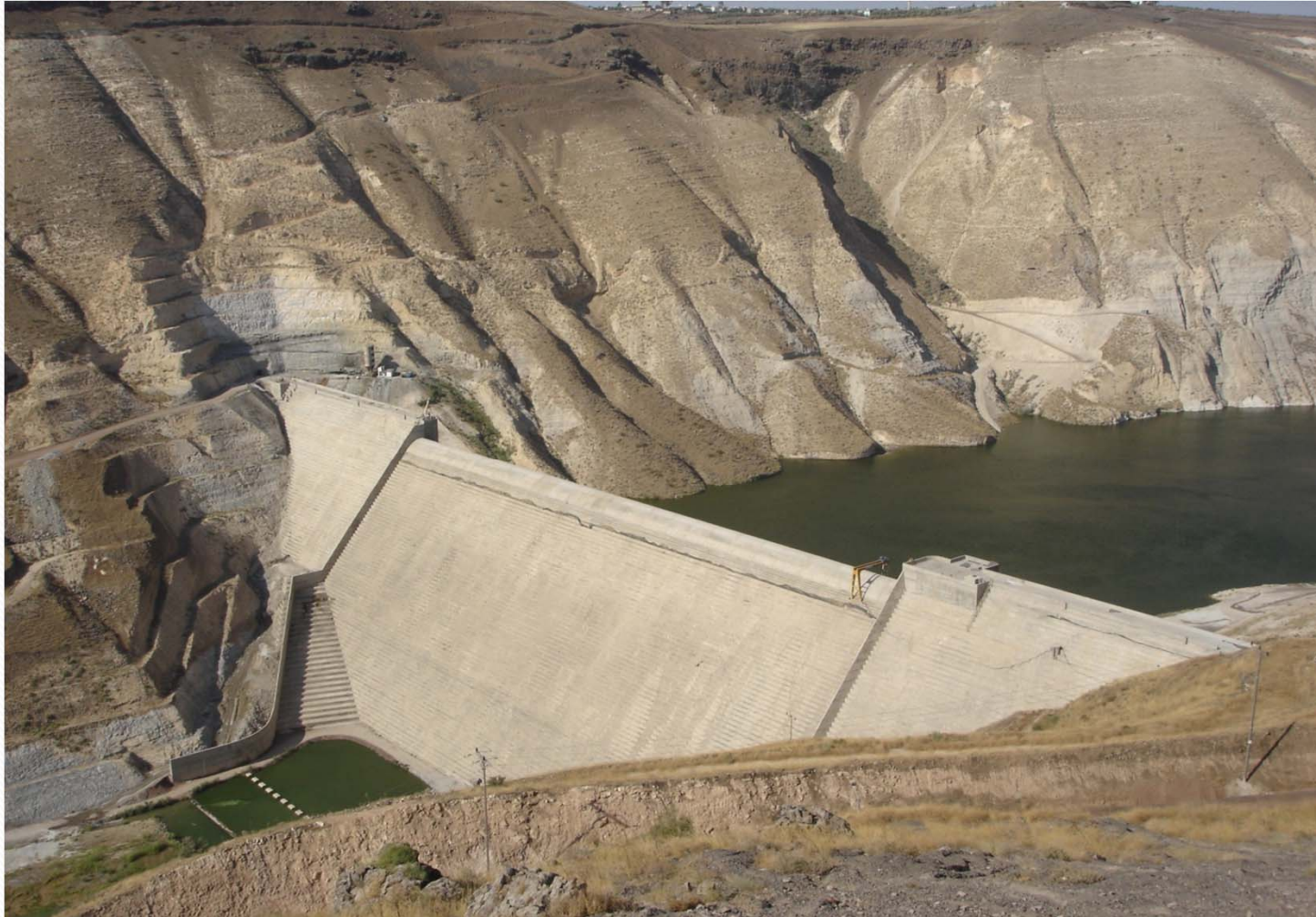
Example of a Roller Compacted Concrete (RCC) dam
