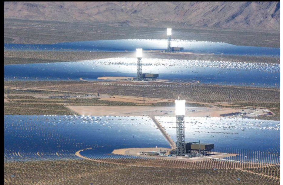
Ivanpah Solar Facility (2016)
